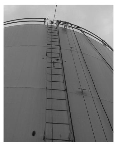
is connected to the cable and the slide is hooked onto a climber's harness. Ladder guards prevent intruders from easily accessing the tank. Round ladder rungs don't offer an edge or grip of any kind, but anti-skid rungs do. They must also be at least 16" wide and should have anti-skid rungs to prevent slips and trips.
